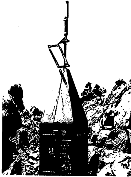
Figure 7.12 National Park Service radio communications repeater atop 3186-m-high (10,453-ft) volcanic Lassen Peak in California. Before installation of the solar panel, a helicopter had to deliver charged storage batteries to the site every two months.
