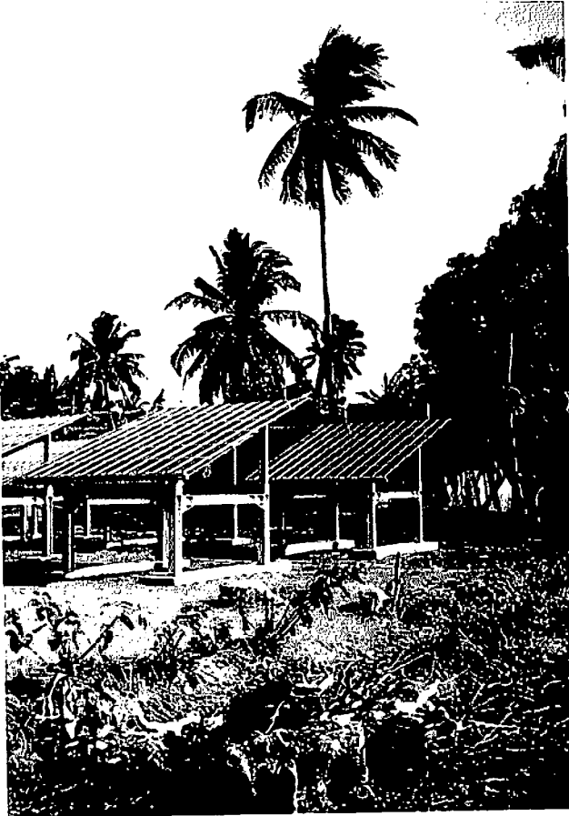
Figure 7.7 Solar cell power supply located in Indonesia. ( Courtesy AEG-Telefunken, with permission. )
